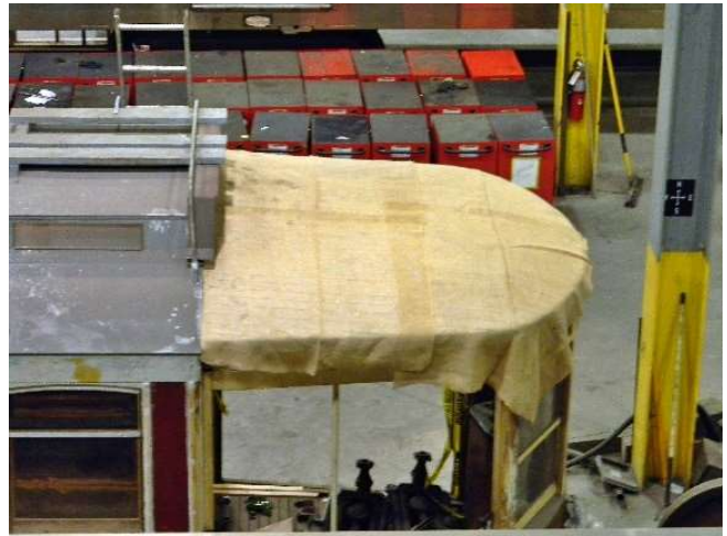
Underlayment is in place.
