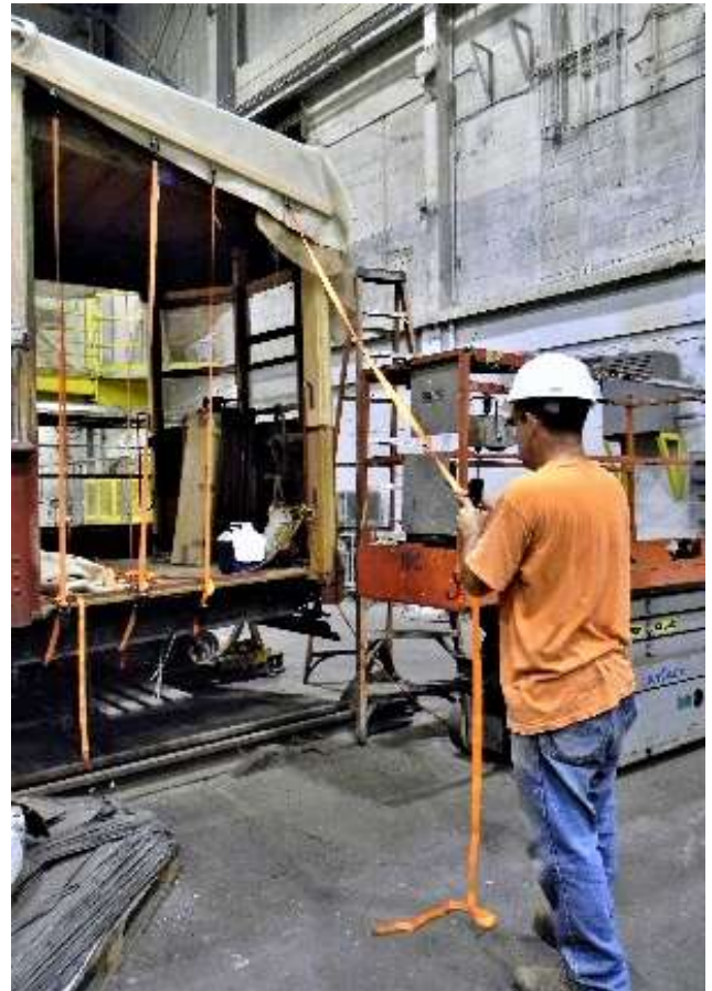
Marc tests one of the ratchet straps, drawing tension on the canvas to remove wrinkles from the roof covering.)
