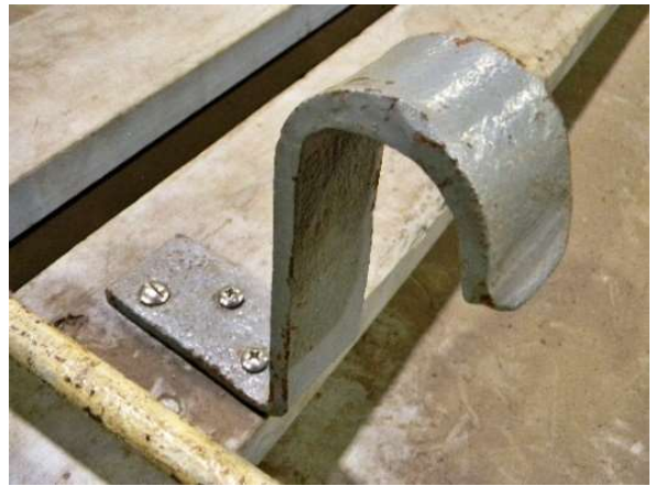
Re-installing both trolley pole hooks presented somewhat less of a problem.
