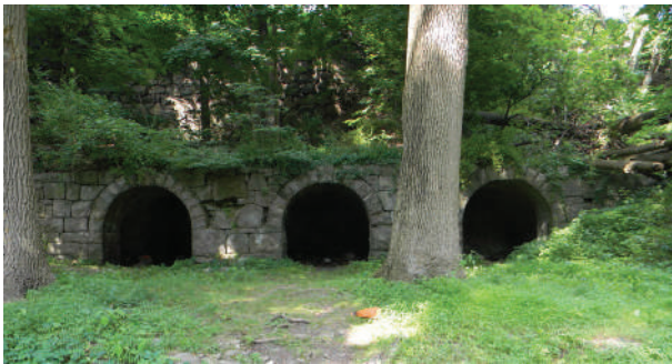
Figure 98: These remains of the Boonton Iron Works provide some mystery as to their specific function. Photo: DSCN3414
