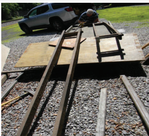
Figure 77: The lifting beam assemblies are winched onto Bob's trailer for moving to the Storage Trailer. Photo: DSCN3405
