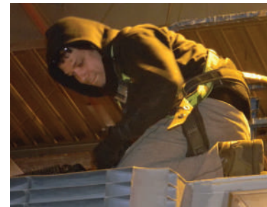
Figure 84: Esteban intently places the bolts to secure the first pole base. Photo: DSCN3300
