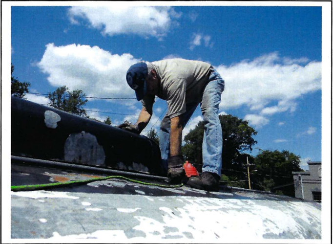
↑With a gorgeous autumn sky as a back drop, Bob begins the removal of the cowl fairing which protects the multiple inlets to the ventilation system as well as the trolley pole.
