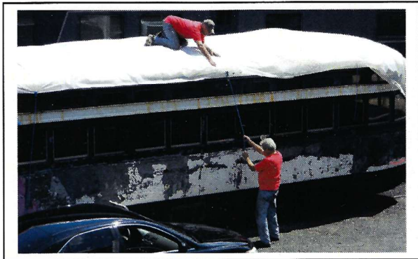
Bob, seen here on the ground, installs and adjusts the many bungee cords deployed to discourage the tarp from becoming a sail.
