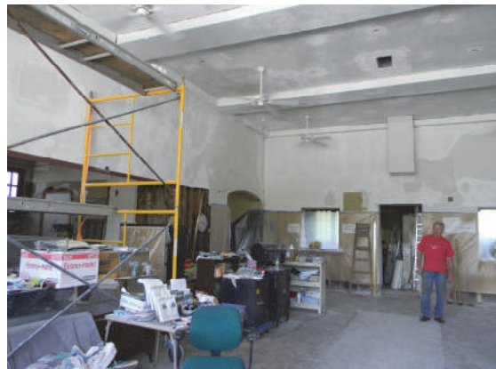
Bob Hooper inspects the freshly plastered ceiling.
