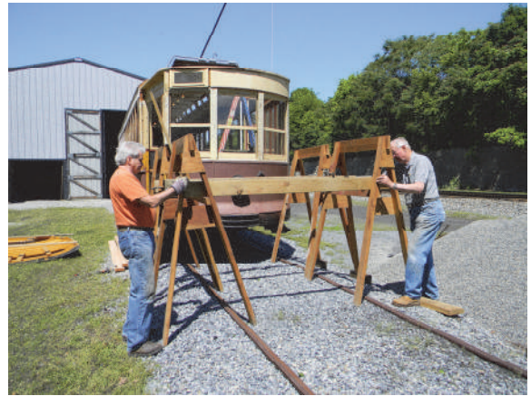
#2 Start by building a trestle!
