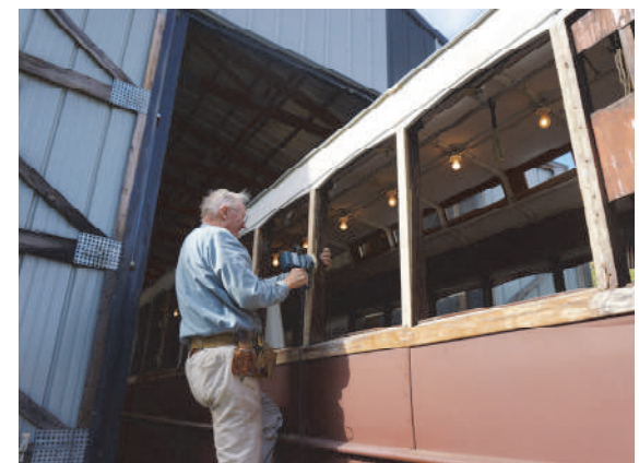
Hank Kaminski works at finishing the window posts.
