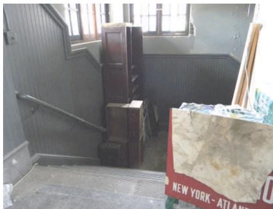
The ticket cabinet temporarily occupies the landing of the DL&W side stairs.
