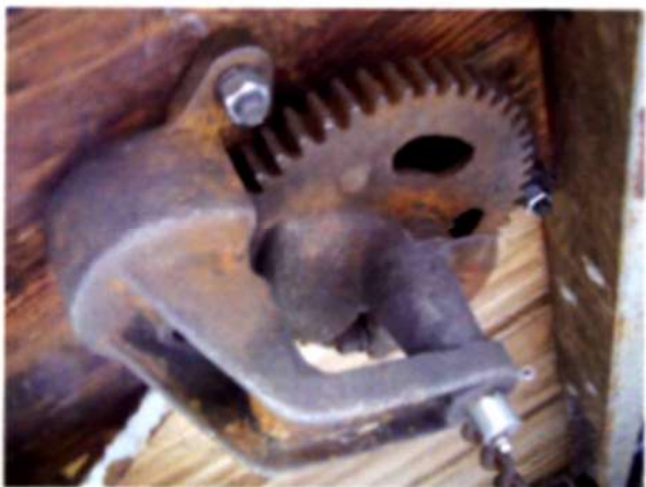
Winder is now held by permanent bolts through platform deck.
