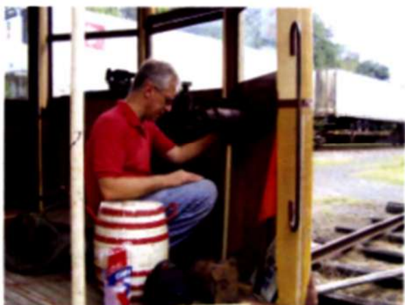
Wooden pattern is made so that a permanent steel torque shaft can be machined to connect the brake wheel gear box with the winder. In the background, NS hustles 100 or more trailers to market.
