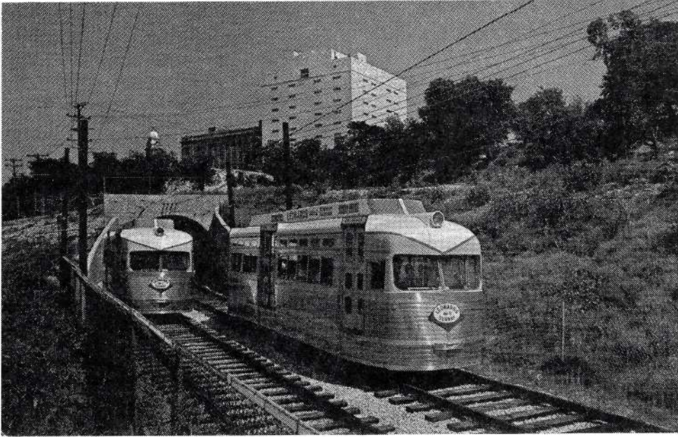
This postcard was published shortly after the Fort Worth subway was opened. It shows two PCC cars in their original standee-window configuration passing at the subway portal.
