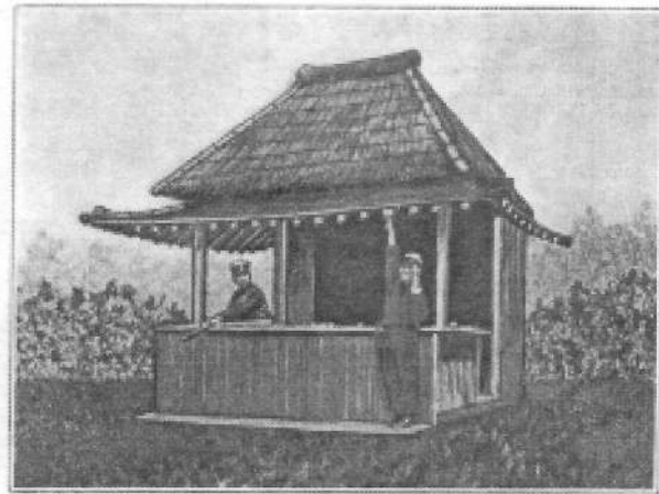
ONE OF THE JAPANESE BUILDINGS UNDER CONSTRUCTION
