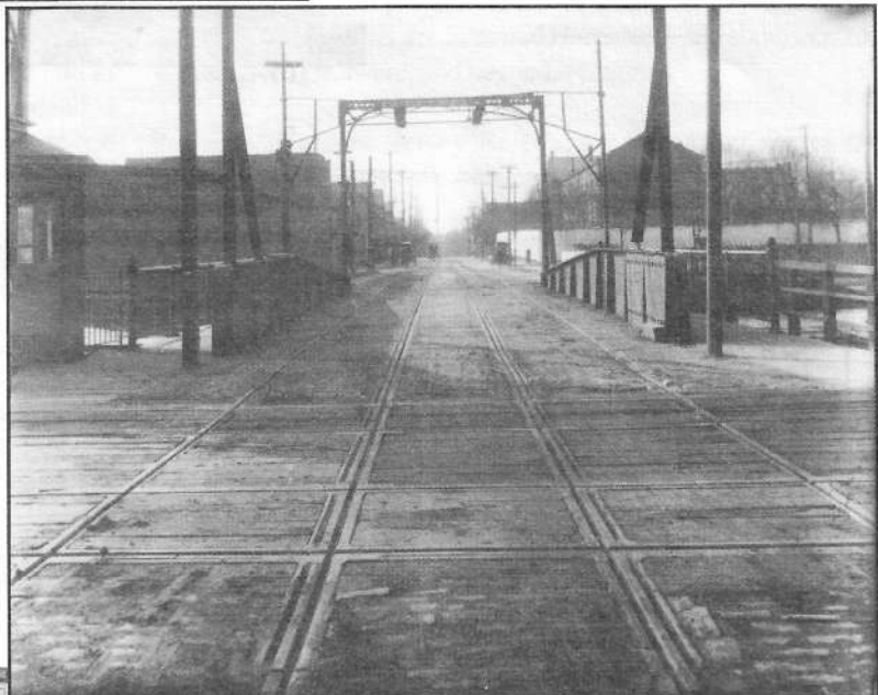
Cass St. & PRR. Crossing - Trenton, NJ - Looking east from bridge over Delaware & Raritan Canal. Double tracked dual gauged trolley line crossed the double tracked PRR Bordentown Branch running along the Canal making for a very interesting crossing. Friends of the NJ Transportation Heritage Center has preserved a similar multi-gauge crossing from the west side of the canal where a freight spur constructed in the 1930s crossed Cass St.
