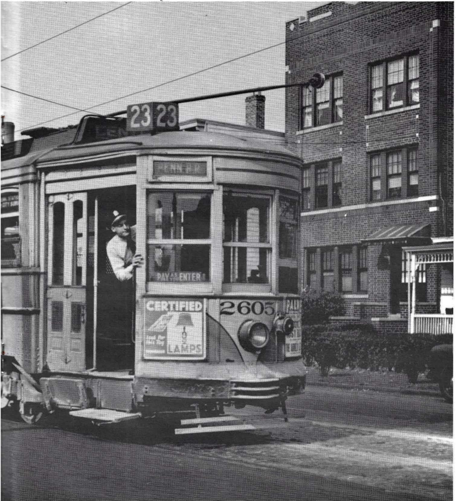
Dick Young photograph Van Buskirk Collection NJERHS Public Service 2605 ready for a run to "Penn Station" October 26, 1947. Photographer Dick Young caught both monitor roof (2605) and deck roof (3212) cars at the end of the 23 Central Line, Central Avenue, Orange, NJ.
