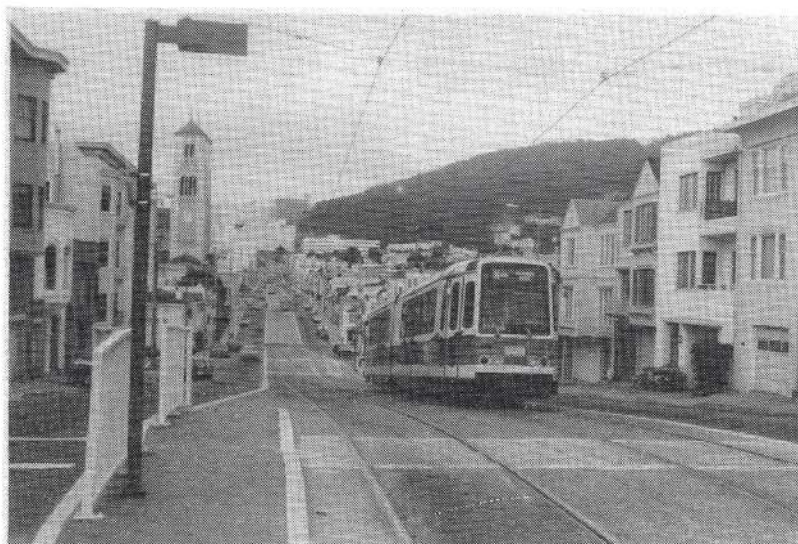
Plans for upgrading San Francisco's streetcar system called for rebuilding most of the street trackage onto raised reservations. Only this short section of Judah Street received that treatment. Further construction of this type was halted in response to the objections of motorists. Frank S. Miklos
