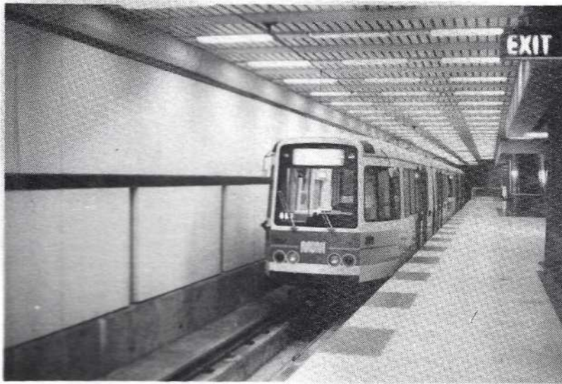
LRVs were tested in the Market Street subway prior to the opening of that facility. This view shows the Civic Center Station at Eighth and Market Streets. Note the raised foundations for the tracks, a reminder of earlier plans for the operation of rapid transit trains.
