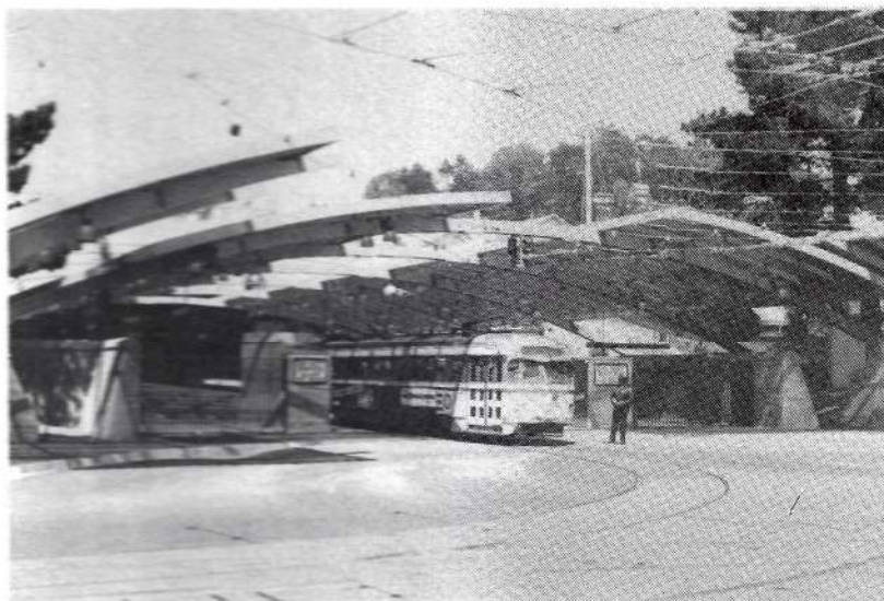
The new West Portal Station has a graceful design that blends in well with the surrounding community. One of MUNI's double-ended PCCs is shown leaving this facility shortly before it opened to LRV service. Frank S. Miklos
