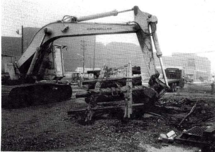
A backhoe raises the Cass Street grade crossing so that it can be loaded onto the truck in the background. This view shows the single railroad track with inbound and outbound dual-gauge trolley tracks crossing at right angles. photo by Bill Christian
