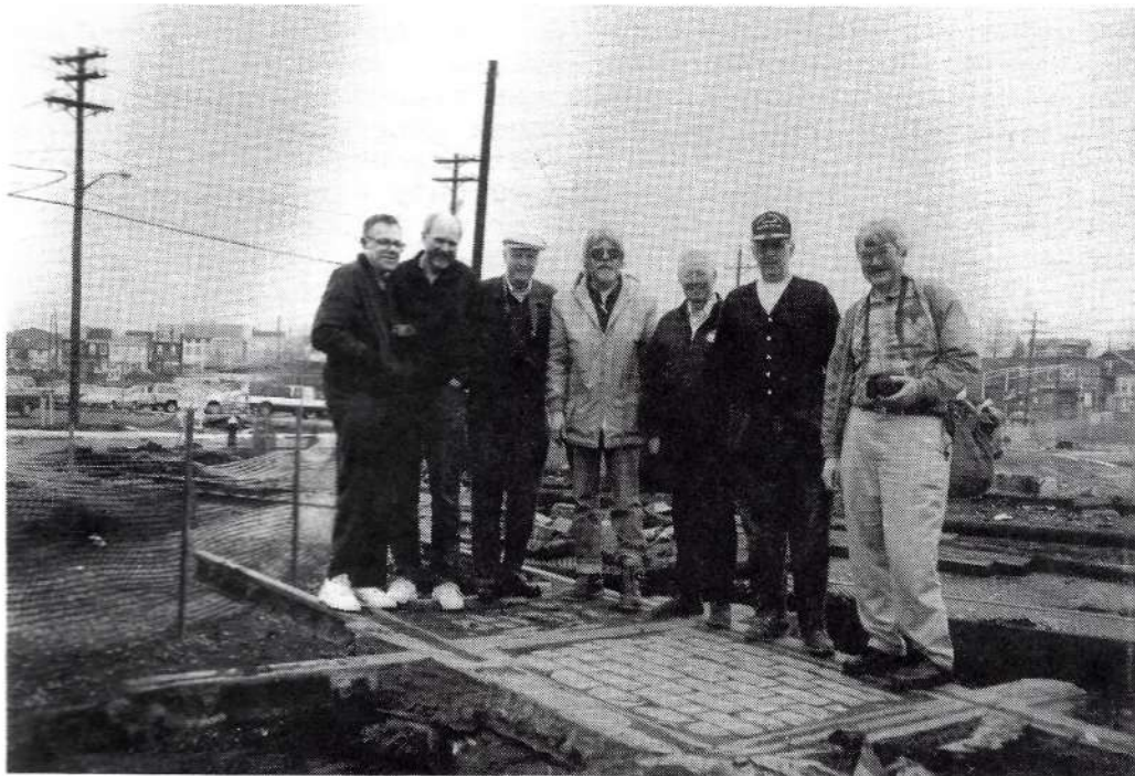
Posing on the recently removed Cass Street grade crossing are Barker Gummere, Gary Kleinedler, Elmer Fry, Bob Yuell, Bill Christian and Frank Miklos. The dual-gauge trolley rails are clearly visible in the lower right hand portion of the picture. photo courtesy of Bob Yuell
